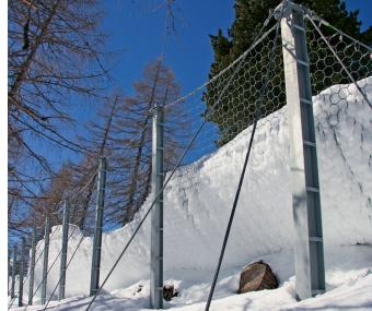
Avalanche protection systems are designed on a site-to-site basis to protect infrastructure, utilities, buildings, reforestation, and lives from avalanches. Unlike other mitigation methods such as control through triggering with explosives, these static defence structures help to prevent snow avalanches from starting in their first stage of occurrence.
