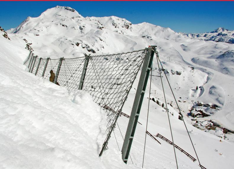
Snow nets prevent the development of avalanches by giving structural support to the snow mass in initiation zones having medium to large snow depths. This is in contrast to other approaches such as artificial release methods - e.g. using explosives – that initiate smaller avalanches before the hazard grows to an unmanageable size.
