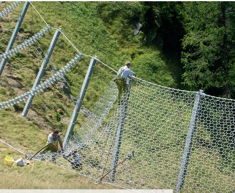
After aligning the posts and installing the suspension and retention ropes, Omega-Nets are pulled open like a curtain and connected together with shackles. Posts and base plates of a snow net system with ball joint - coupling on the post foot and ball on a base plate. Saddle plate with the mounting tube on the post head for easy net installation.
