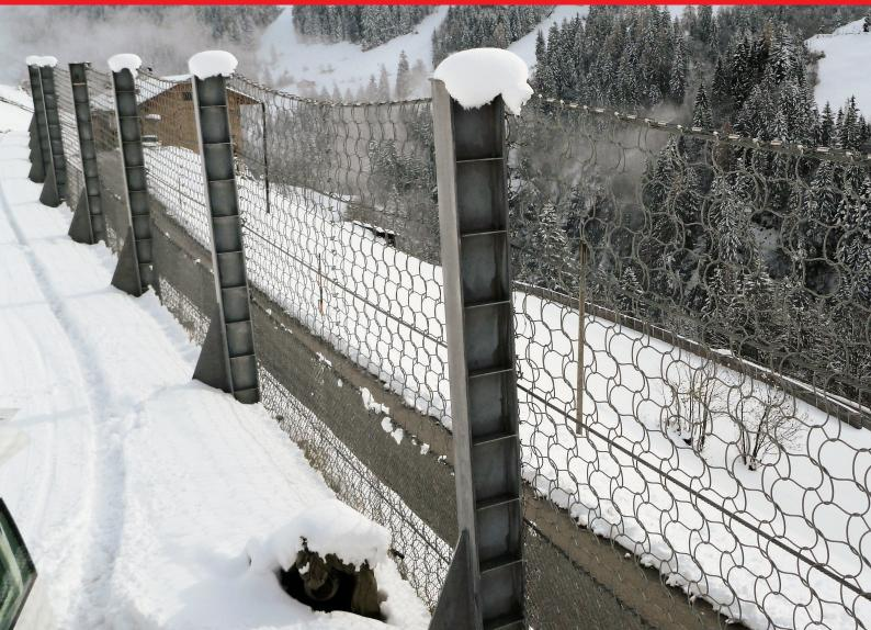
Snow catchment fences such as the SNOW-CATCHER do not prevent the initiation of avalanches but instead interact with an avalanche in the run-out or deposition zones, to slow the avalanche and bring it to a standstill. This shortens the destructive reach of avalanches.
